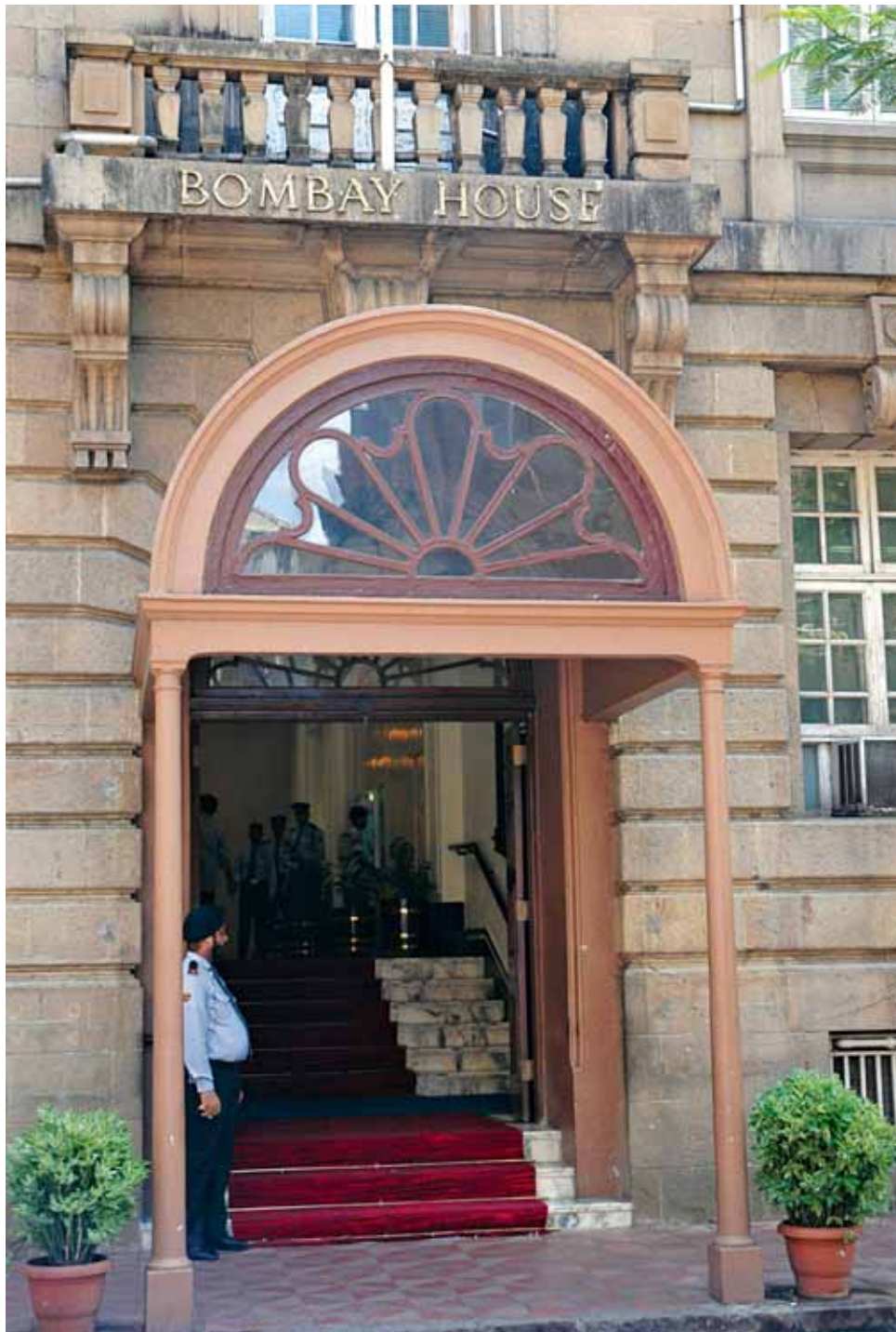
Bombay House, headquarters of Tata group.
